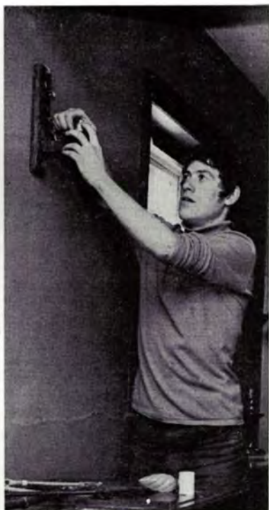
Electrician Gareth M. Joseph makes the final connections to the cooker control unit in the all-electric kitchen in the hotel.
