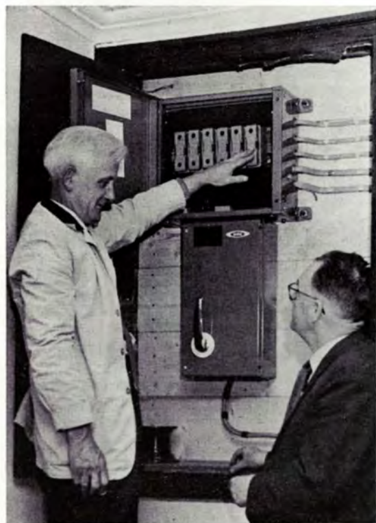
Mr. George Davies ( foreman electrician ) left, discusses a point on the installation with Mr. Walter Williams ( consumers' engineer ).
