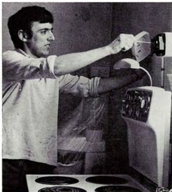
Electrician Gareth M. Joseph makes the final connections to the cooker control unit in the all-electric kitchen in the hotel.
